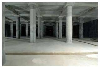
Photo 3.4 Underground Stormwater Storage Facility Beneath Sanno Park, Fukuoka City
