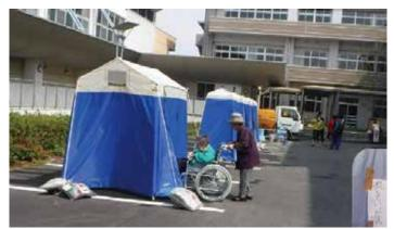
Photo 3.12 Manhole Toilets Used in Kumamoto City after 2016 Earthquake
