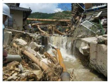
Photo 3.7 Exposed Distribution Mains in Asaminami District after 2014 Landslides in Hiroshima
