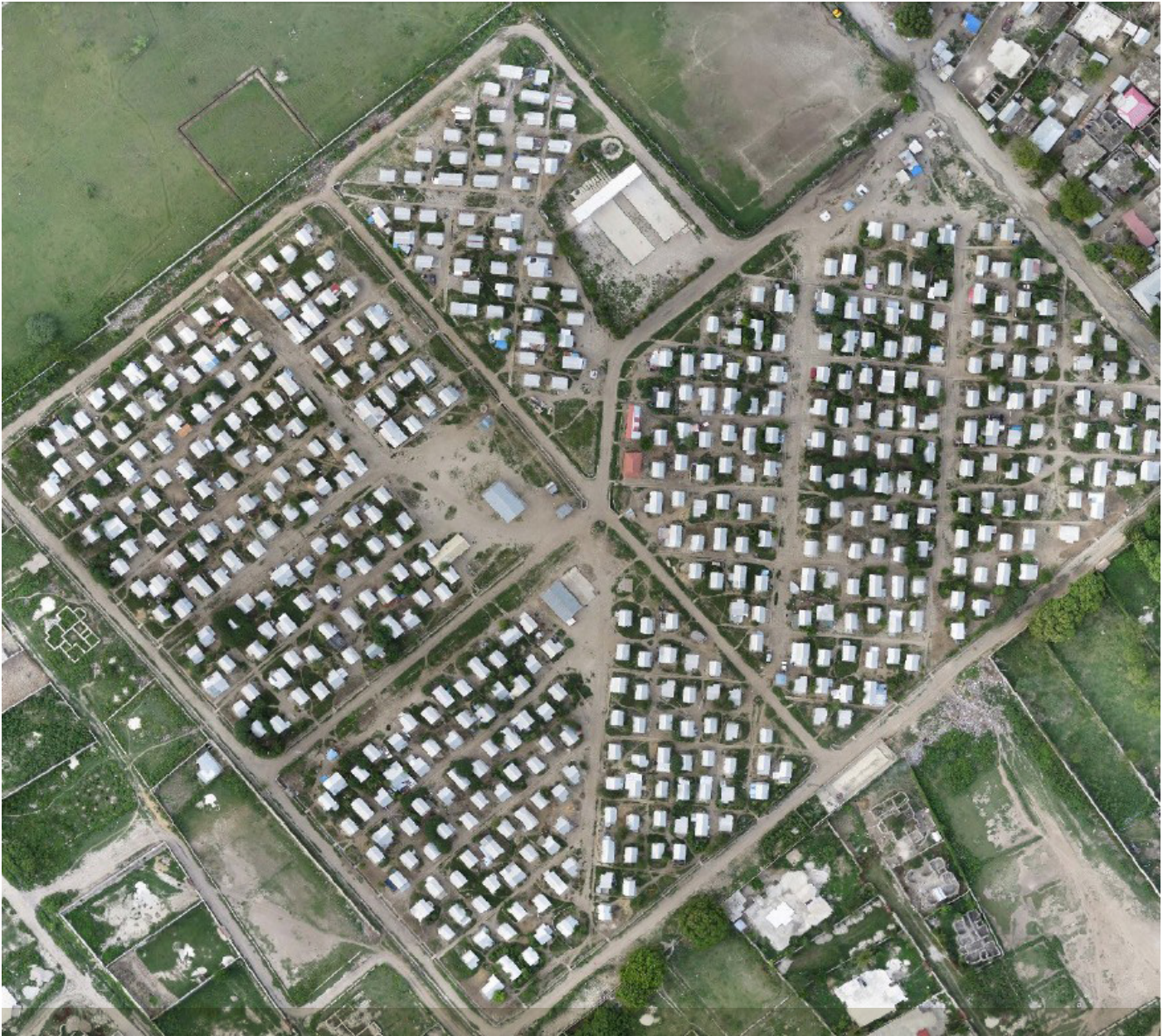
Figure 4 Up-to-date imagery and an elevation model allowed the shelter unit to plan new construction effectively
